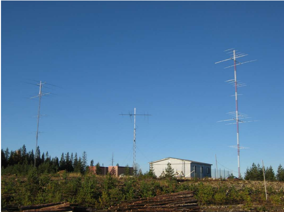
10-15-20-40 Yagis, WRTC-beam, Shack, 105-m tower.
