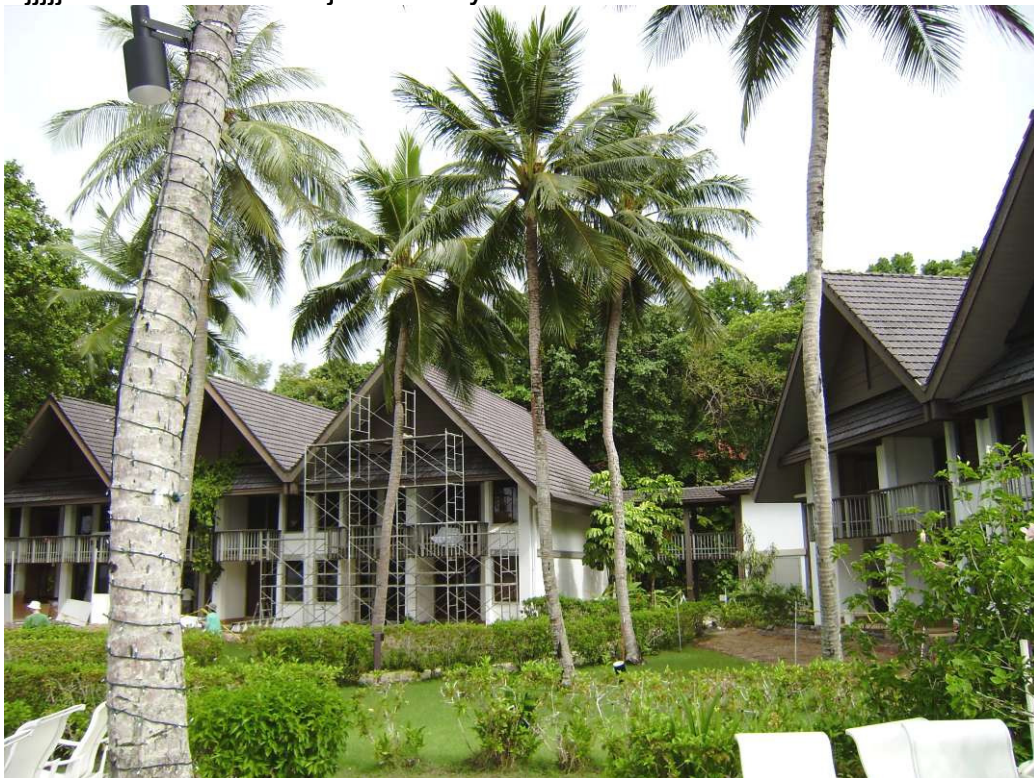
The QTH under renovation.
