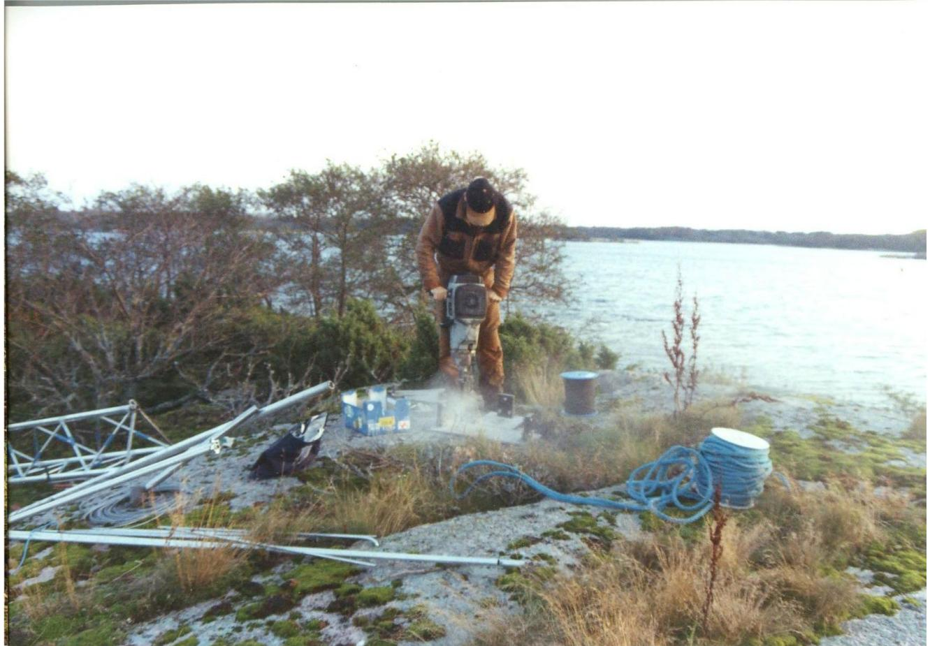
Pekka, OH7RM (see PileUP! 12(4)) using OH2AQ's drill for the 160/80M aluminium-mast, which had a total length of 30 M, and tuning for 160M was done with a linear loading.
