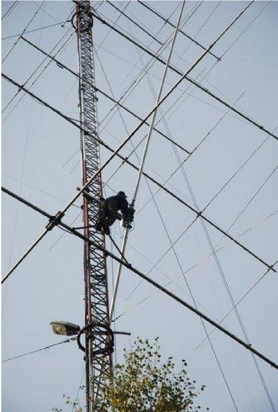
Lifting the lower dipole to 22 meters. (Photo OH2JA)
