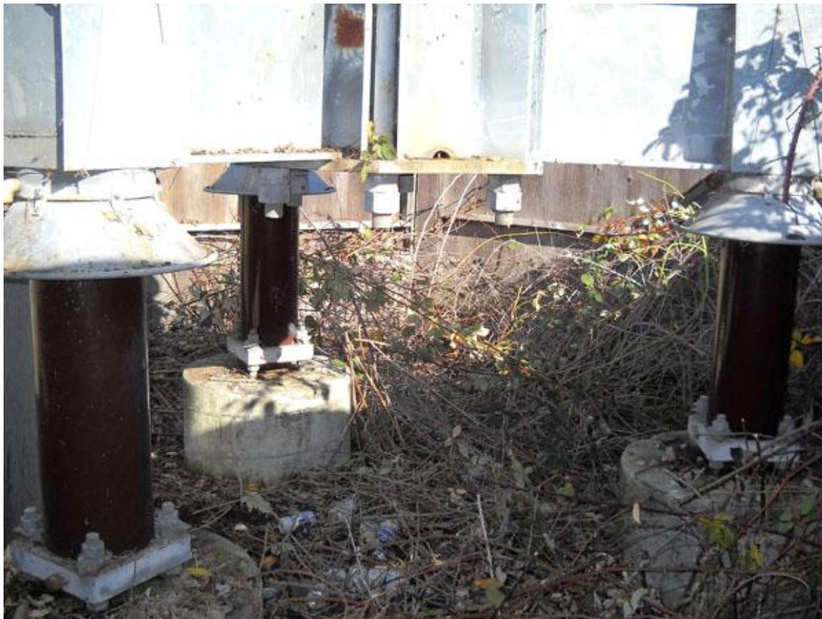
**Fig. 2.** Three adequate insulators at the base of each flagpole antenna. Notice the wild vine growing around.
