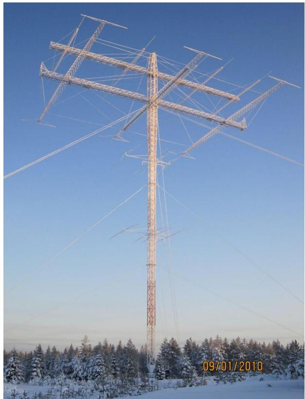
M7 in the -30C frost with the new 40m 4o4 and enforced base section.
