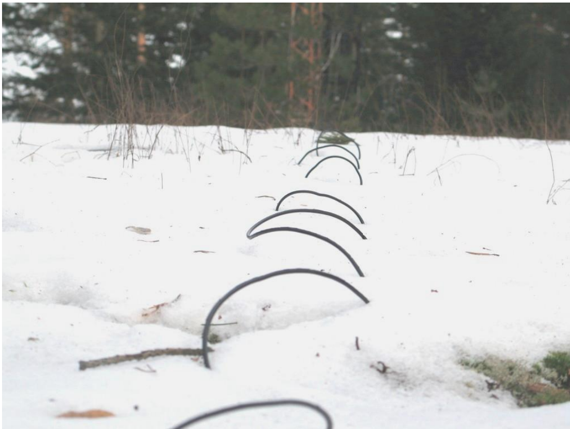
Helix-radials @ OH5Z. Their impact is ca. +6dB. Patent is pending. (OH1WZ)
