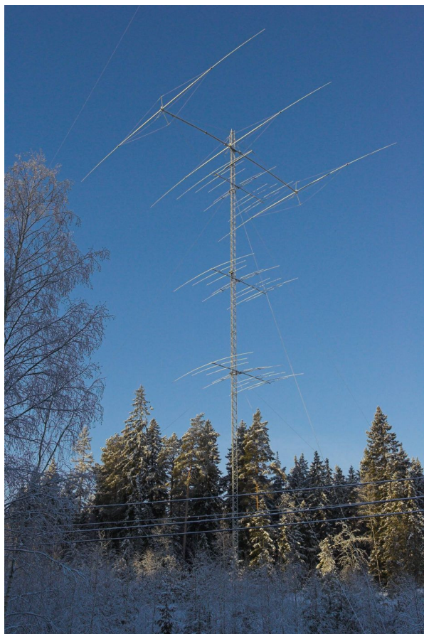
Figure 4. The 48-meter tower with the K6MYC-beam up at the top. The other 3 antennas make a stacked array of tribanders for 14-28 MHz. Photo OH2BH.
