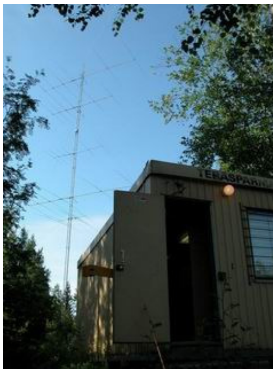
Figure 5. The shack, a container with one of the 42-m rotatable towers in the background. Photo ON4UN.
